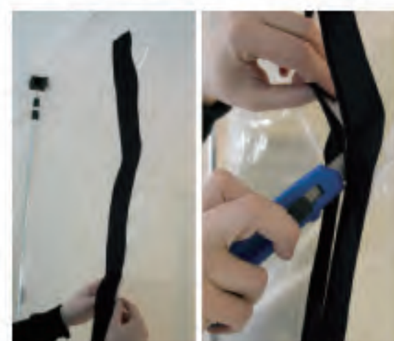
6. To create an access: apply the adhesive zipper, open and cut the sheet following the zipper.
