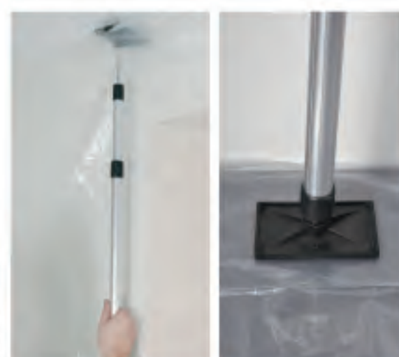
3. Raise the pole with spring loaded head against the ceiling. Start at either side.
