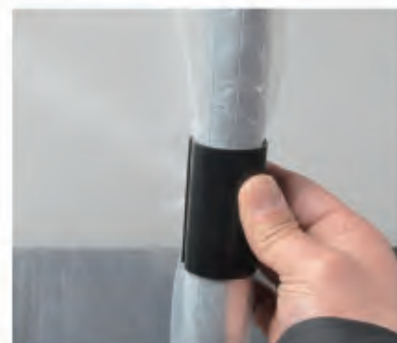
5. Secure the sheet vertically with the U-clips.
